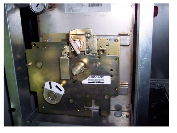
Above a gas filled isolation switch that is placed inside the bottom of the turbine mast, to cessate (cuts) the power when required.
